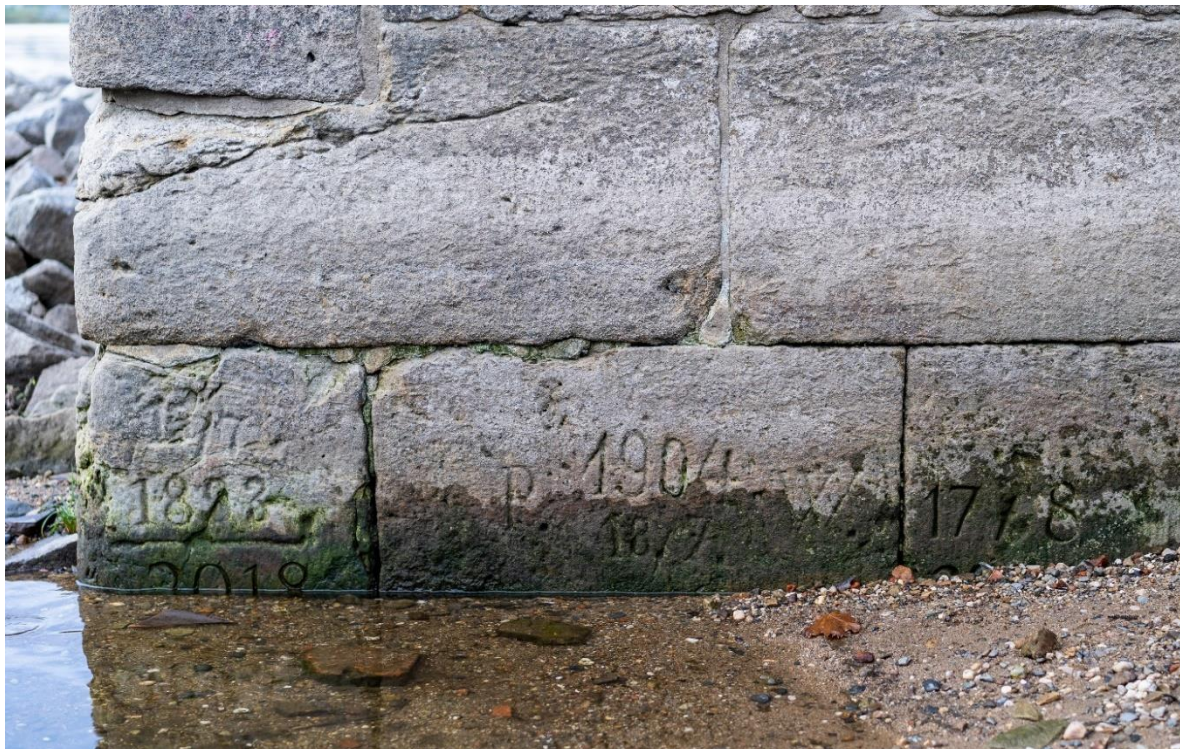
Engraved low water markings, also known as hunger markings. Recent record low year 2018 is still visible. These markings are found at the Elbe river at Pillnitz near Dresden, Germany. Credits: Daniel Albach / Shutterstock
