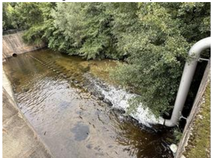
Figure 4: Regenerated water from Figueres wastewater treatment plant returned to the Muga river for ecological flow.
